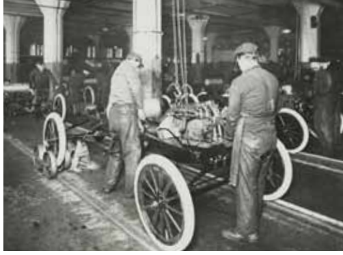
Workers Installing Engines on Ford Model T Assembly Line at Highland Park Plant, 1913
