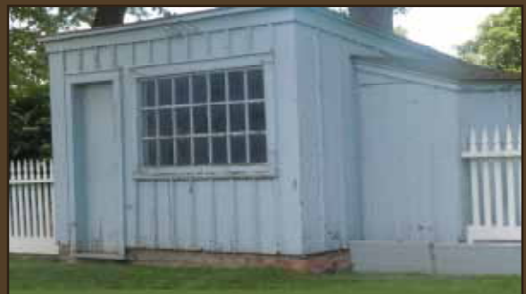
Shed for Preparing Carbon
