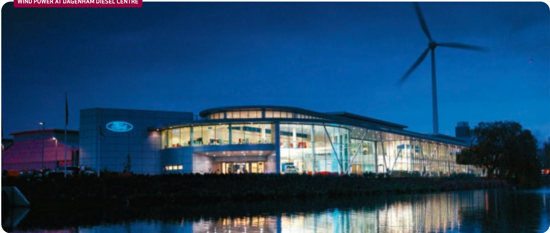
WIND POWER AT DAGENHAM DIESEL CENTRE
