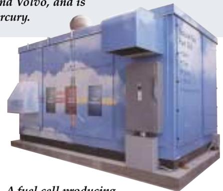
*A fuel cell producing 200 kilowatts of electricity and 900,000 BTUs of heat provides 25 percent of the building’s power.*
