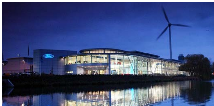
Dagenham Diesel Centre, UK
