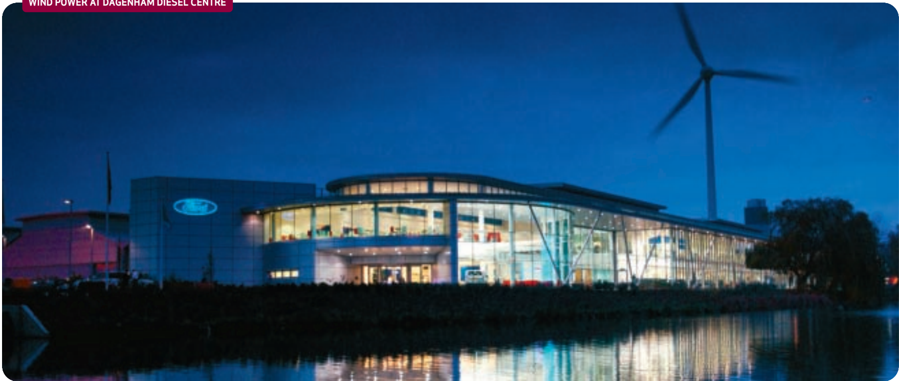
WIND POWER AT DAGENHAM DIESEL CENTRE
