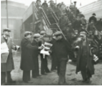
Site of the “Battle of the Overpass” in 1937, the foot bridge at Gate 4 is recognized by the U.S. National Park Service as one of the ten most significant sites in labor history.
