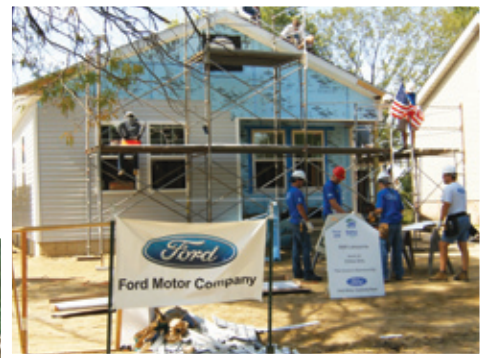
Blitz Build in Detroit, Michigan.
