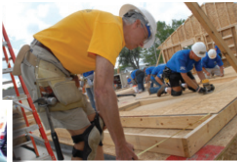
Habitat for Humanity build in Detroit, Michigan.
