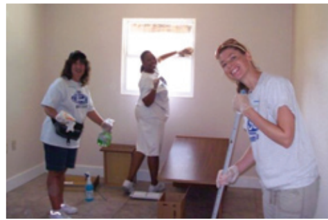
Vacant home rehab in Melbourne, Florida.
