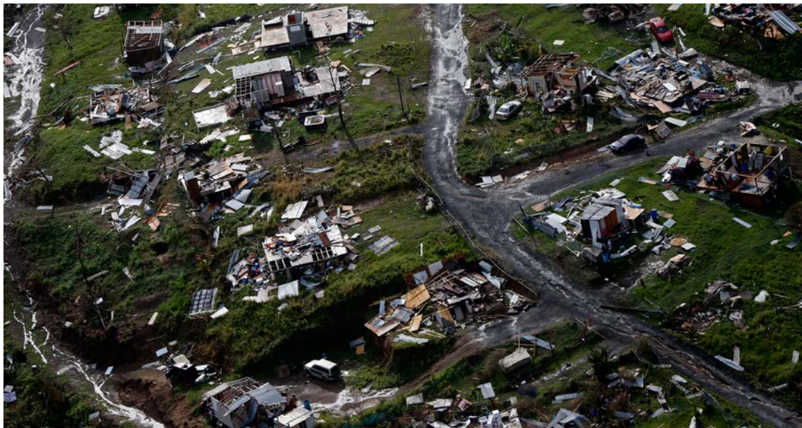
Destroyed communities are seen in the aftermath of Hurricane Maria in Toa Alta, Puerto Rico. (Photo: Gerald Herbert, AP)
